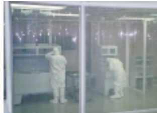
CLASS 1000 CLEAN ROOM
