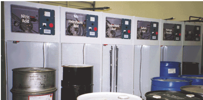
Chemical distribution stations allow bulk chemical delivery to systems on demand or automatically.
